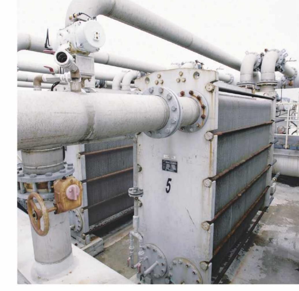
Heat exchange of black liquor / white water, oven blow gas condensation, waste heat recovery
