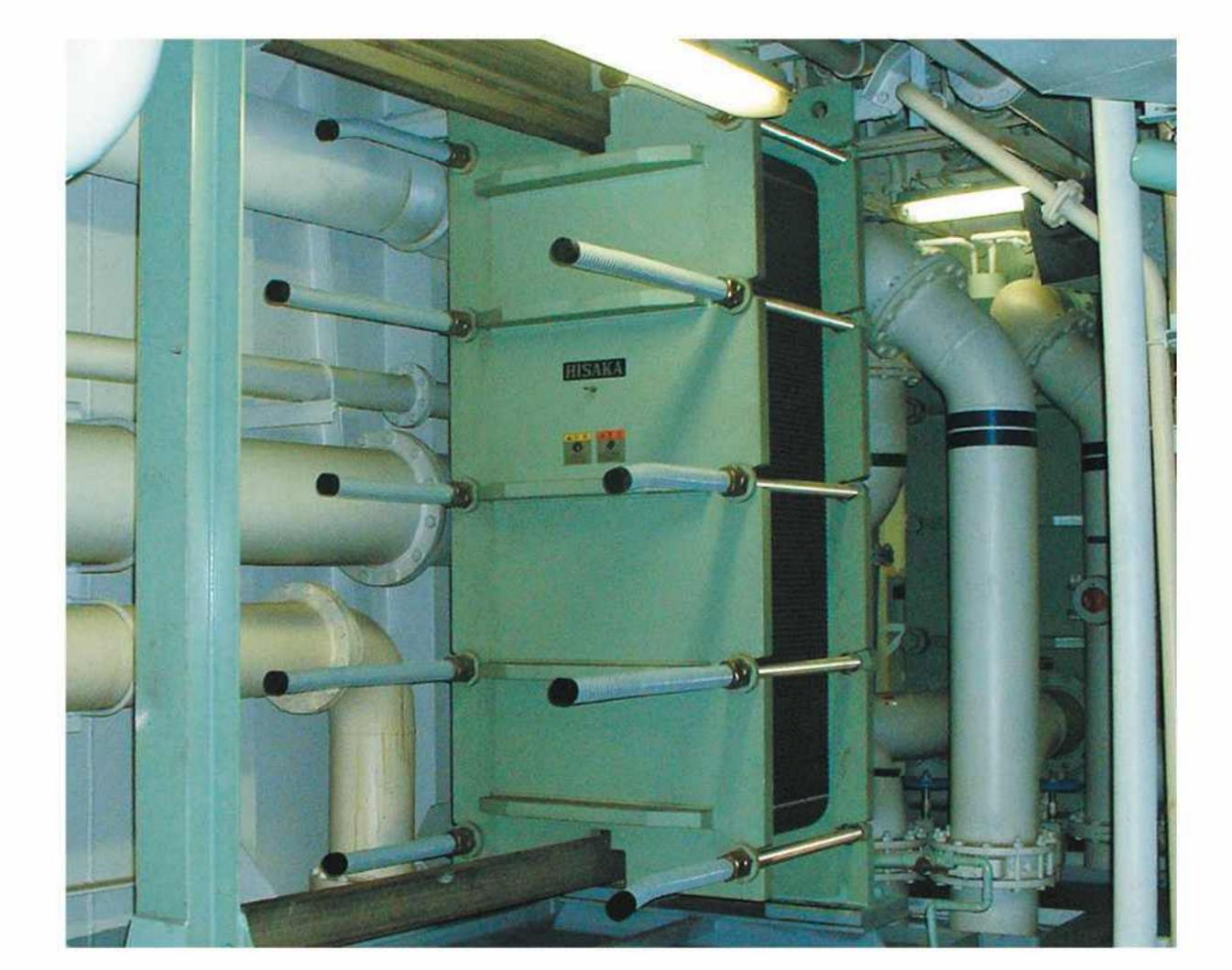
Cooling of engine jacket water and lubricant oil
