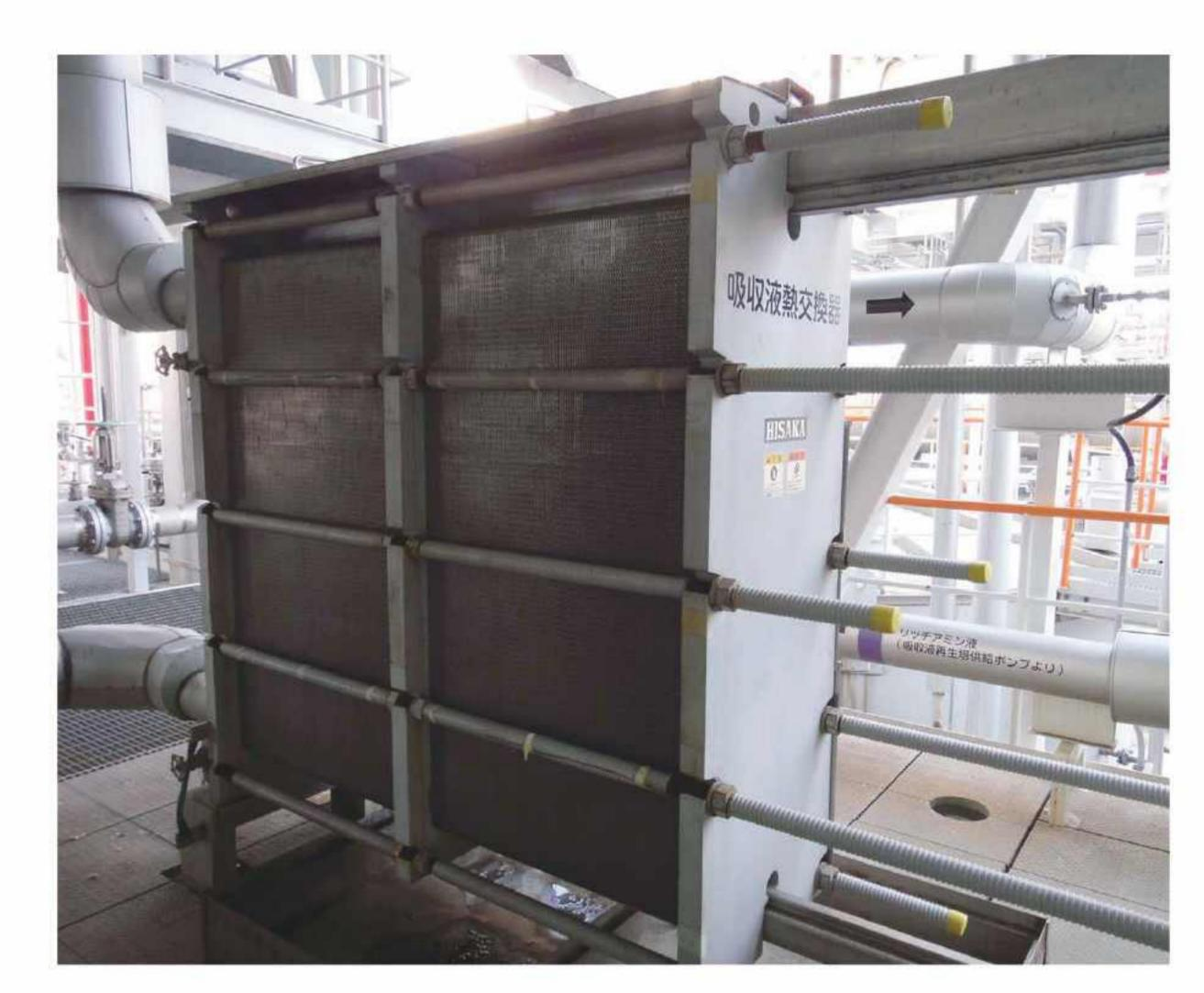
CO2 recovery, desulfurization plant solution heat exchange
