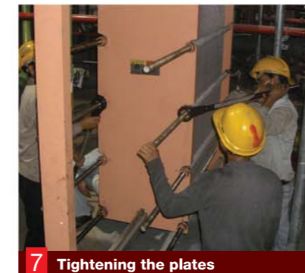
7 Tightening the plates
