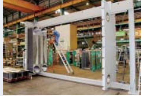
Assembling a large plate type heat exchanger
